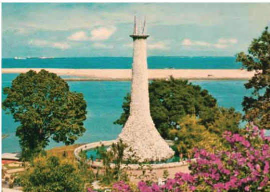
The Coralon tower, mid-1970s National Museum of Singapore Collection, courtesy of National Heritage Board
