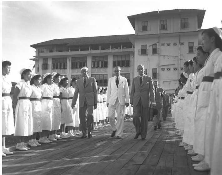
Governor Sir John Nicoll at the foundation stone laying ceremony of Block 1 (of the Former KKH), with Block 2 visible in the background, 6 October 1953. Courtesy of the National Archives of Singapore.
