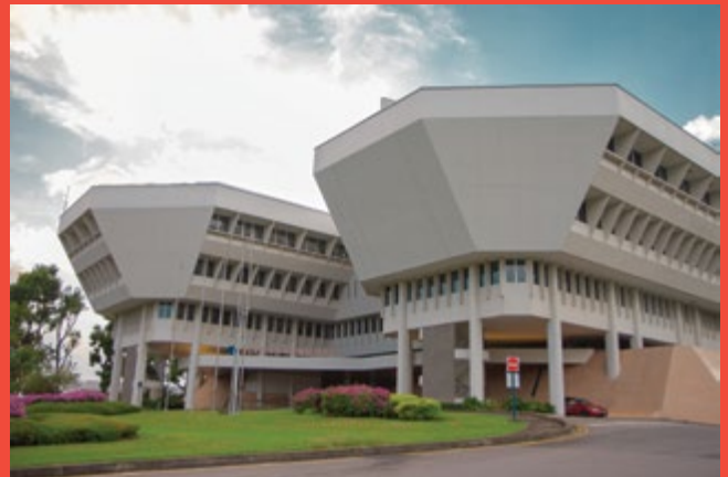
Jurong Town Hall Building
