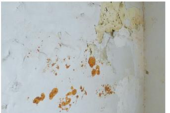
From top: Severe paint blistering on a wall due to the use of incompatible paint (film-forming paint); and plaster spalling, excessive salt accumulation and paint blistering due to moisture trappedbeneaththe film-forming paint of this column pilaster.
