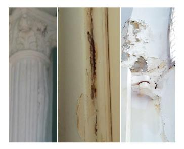
From left: Bulging column caused by trapped dampness within; signs of metal corrosion within damp structure; and spalling plaster and flaking paint.
