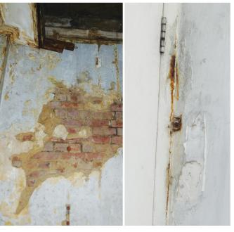
Fron left: Incompatible paint results in severe plaster and paint deterioration; and accumulated dampness within walls causes embeddedmetalbars to corrode.
