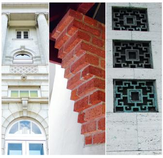
Original finishes that must be retained: (from left) Shanghai plaster finish; facing brick finish; and natural stone finish.
