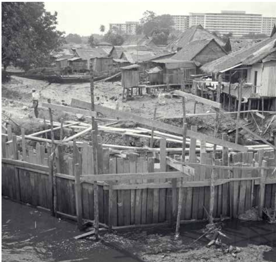
Improvement works along Sungei Kallang at Braddell Road to reduce flooding in Potong Pasir and Toa Payoh, 1968.
