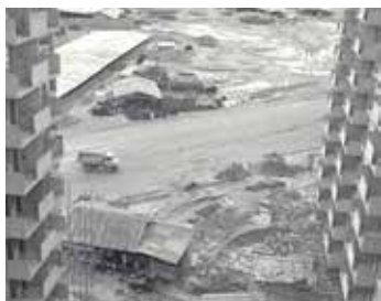
A Housing & Development Board (HDB) estate under construction in Toa Payoh, 1965.
