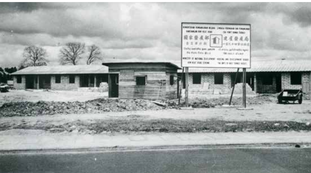
Basic terrace houses being built at Kim Keat Road, 1962.
